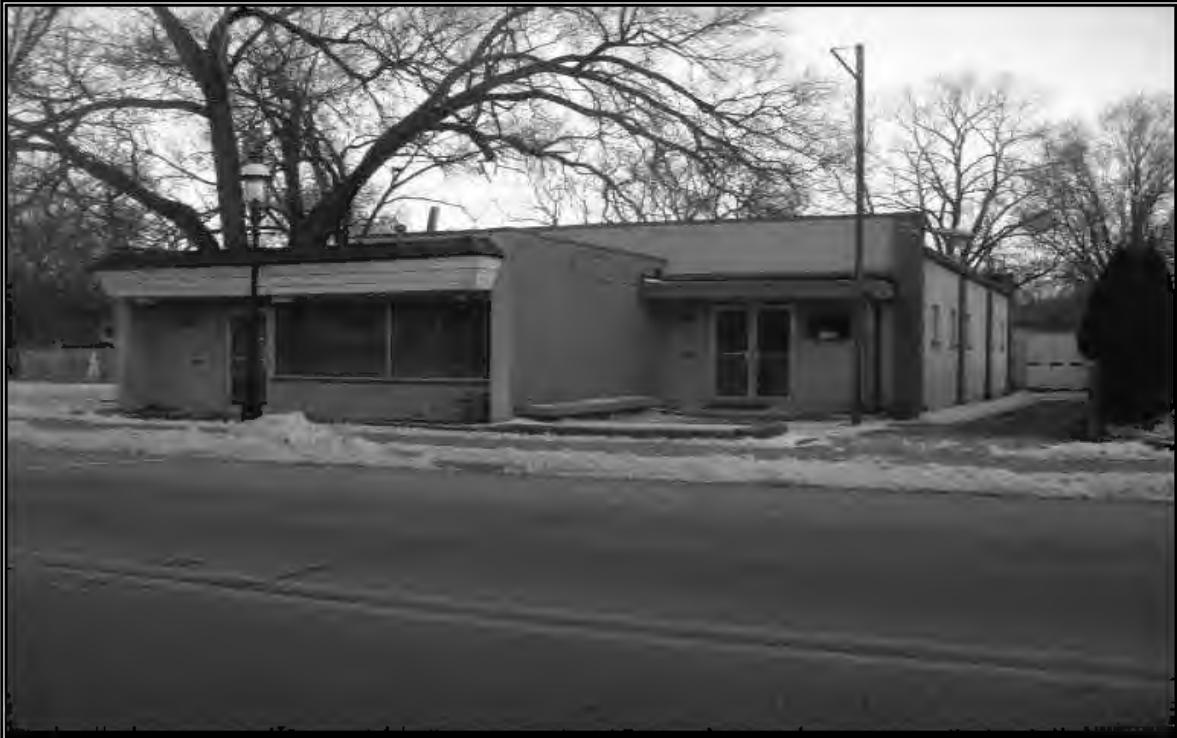
South and East Elevation of Commercial Building
