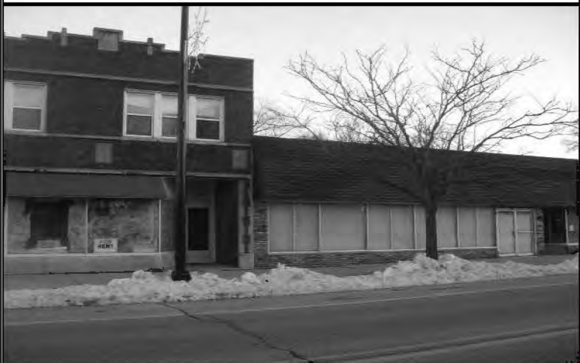
South Elevation of Mixed Use Building and Commercial Building
